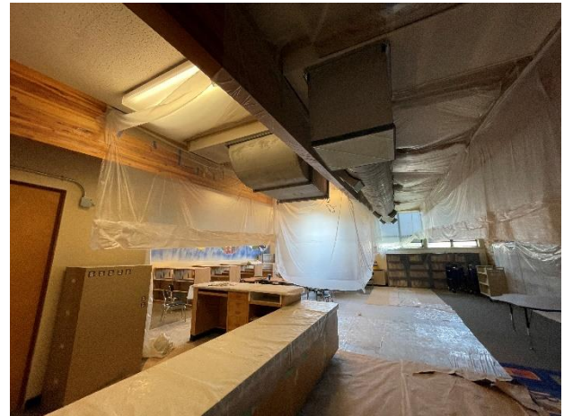
Brooklyn – new ceiling-mounted ductwork taped off and ready for painting.
